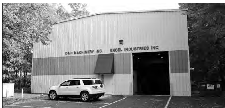
Our Warehouse - 20,000 square foot heated facility with 20 ton crane, located at 1745 Commerce, Holland, Ohio
